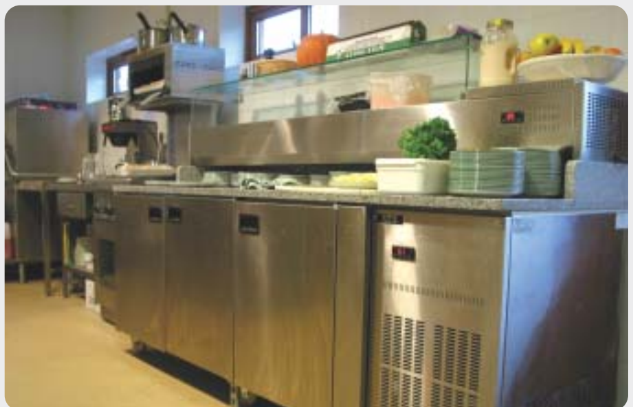
A well-run and maintained kitchen, Llama Centre, Wych Cross
